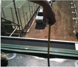
If standing seam roof panels are installed on an out-of-plane roof substrate, there is the potential for improper panel-and-clip engagement at the side laps
